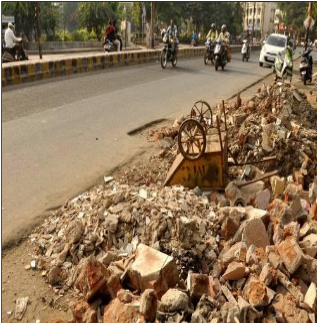
Figure 2.1: Indiscriminate dumping of C & D wastes along roadsides
