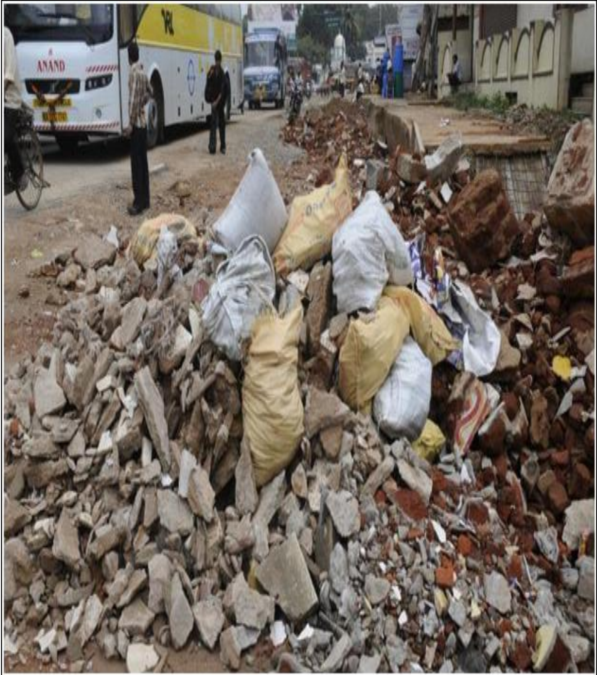
Figure 3.1: Indiscriminate dumping of C & D wastes along roadsides
